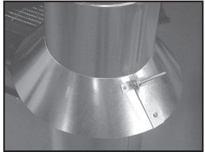
Figure 8.19 Assembling the Storm Collar Around the Pipe
